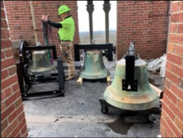
A worker installing the bells at Ferdinand
